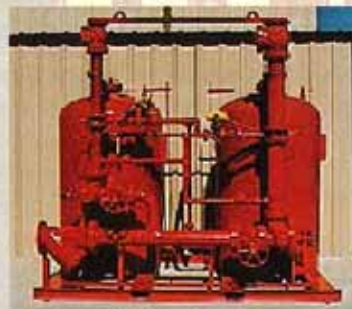
This twin vertical bladder tank system provides both dual and redundant systems capacity depending upon situational needs.
